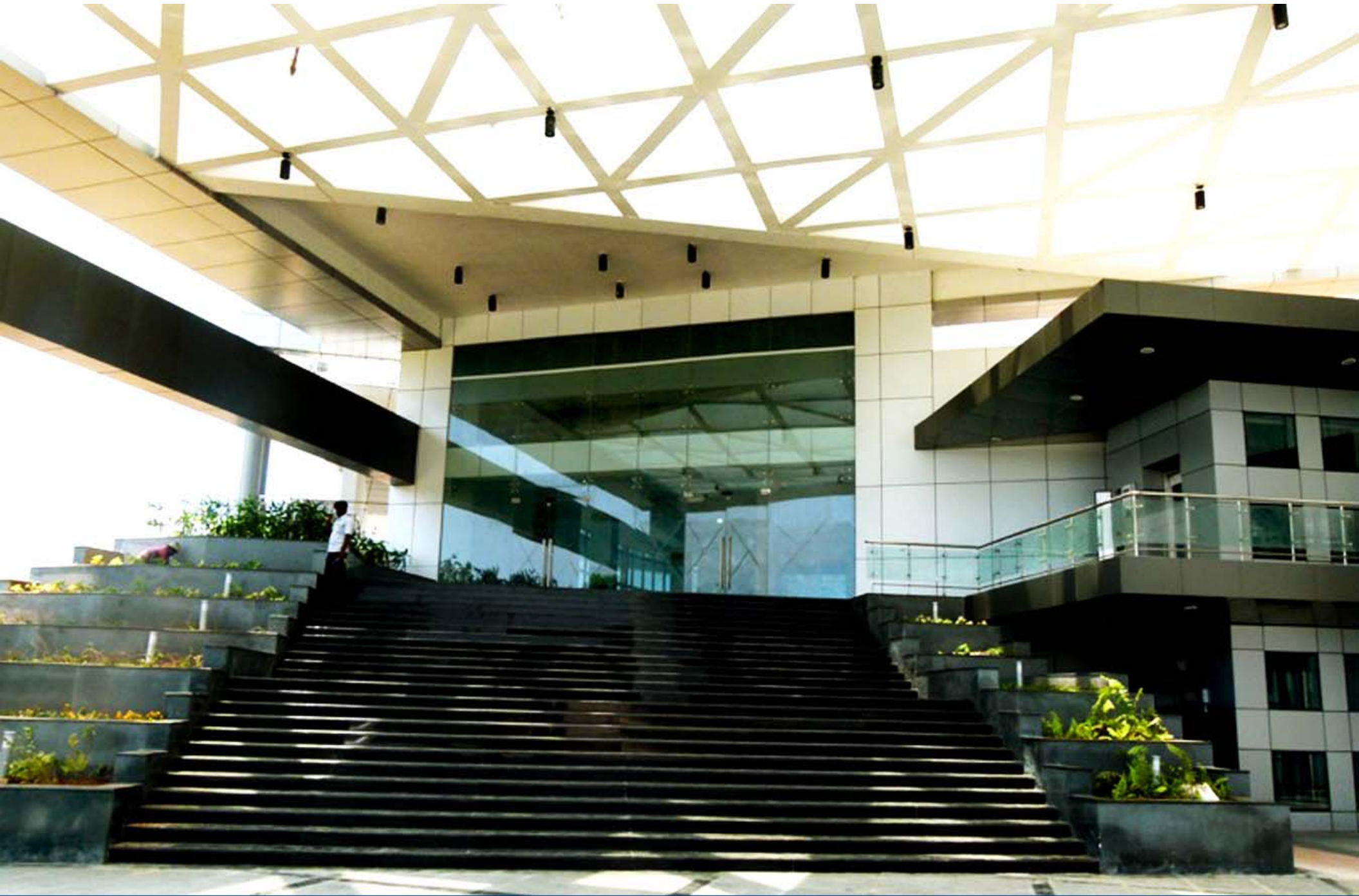
Anna Centenary Library Auditorium Kotturpuram, Chennai
